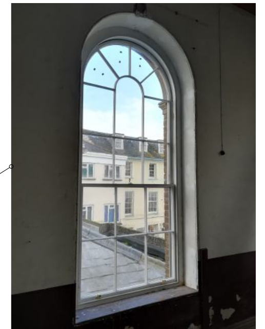
One refurbished window
