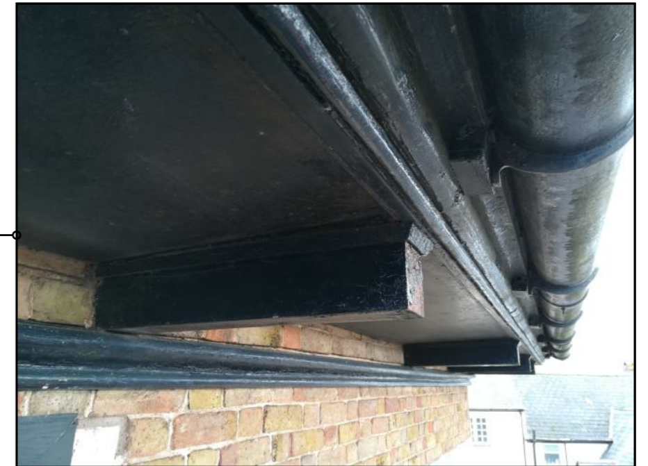
Gutters, fascia and soffit
