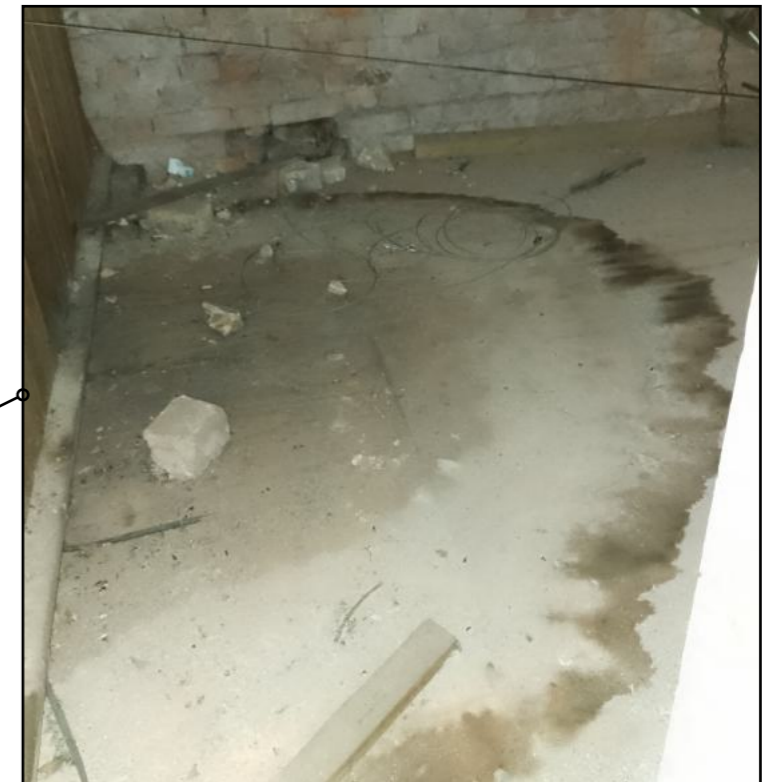
Damp in roof above ceiling of main hall
